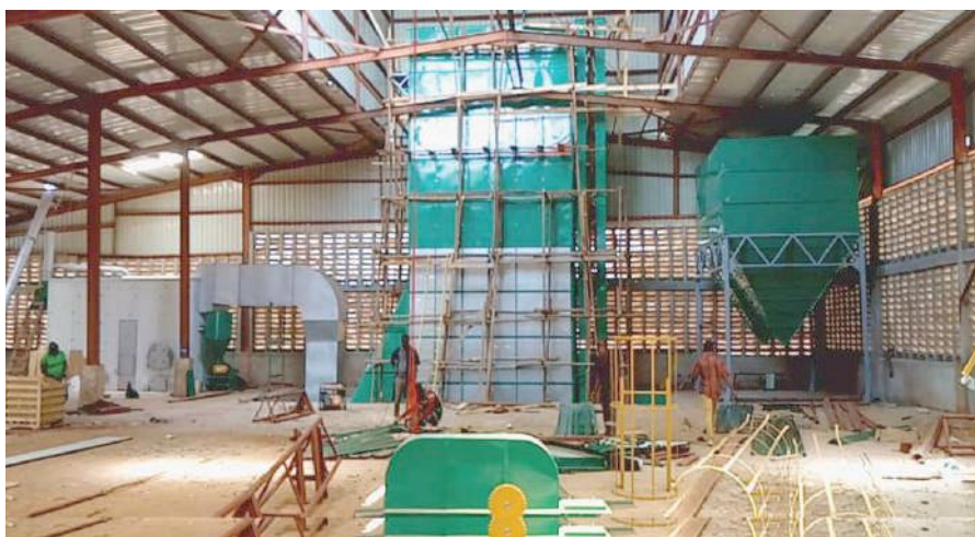
The new 3,150MT mechanical coffee drier in Mbinga that is under construction.
